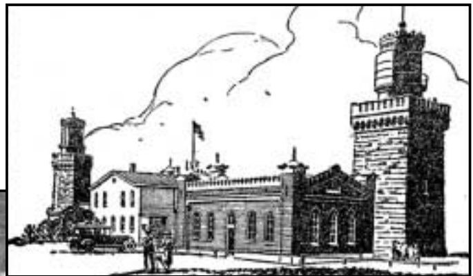
(Above) Twin Lights, Know Your State , 1925. Renowned as "the most powerful light in America," the Navesink light was visible 22 miles at sea. The present building was constructed in 1862. Though called twins, the south tower is square while the north tower is octagonal.
