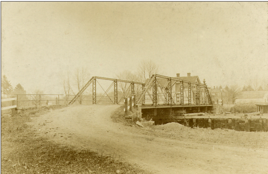
Both photographs of the 1889 bridge taken shortly after it was built.
