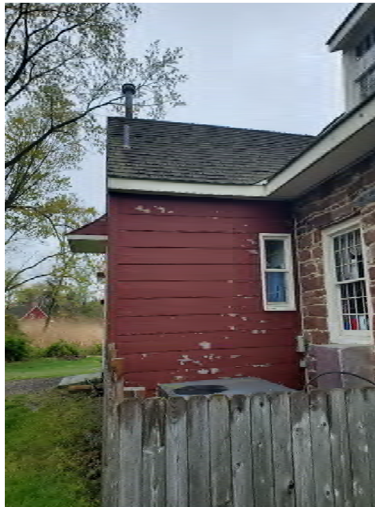
DELAMINATING PAINT
