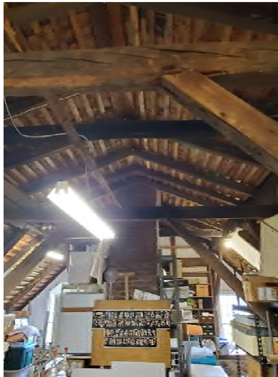
EXISTING STRUCTURE AND OPEN SHEATHING
