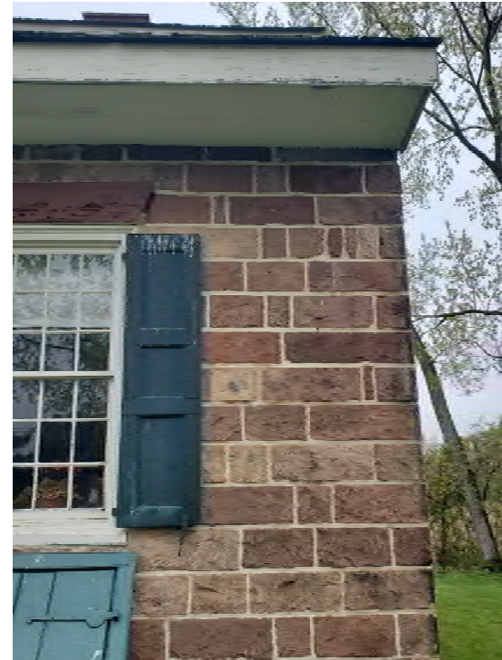
DELAMINATING PAINT AND DETERIORATED WOOD TRIM
