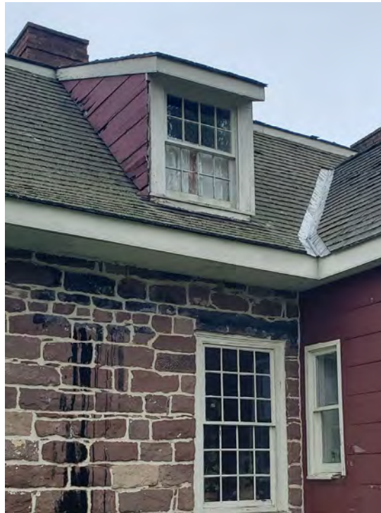
DAMAGED WOOD SIDING
