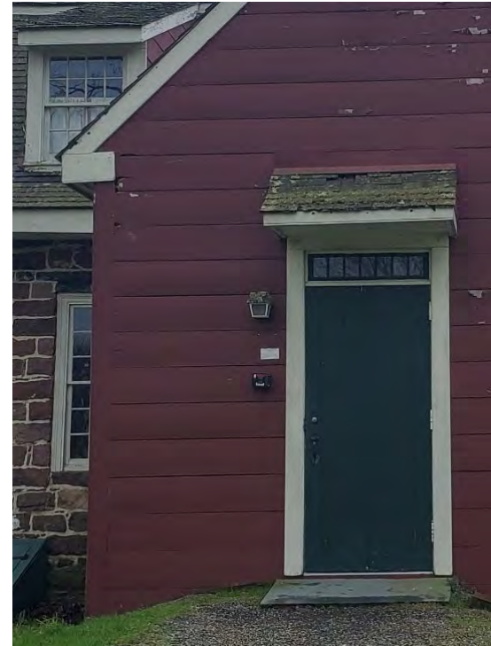
DAMAGED ROOF AND DETERIORATED WOOD TRIM
