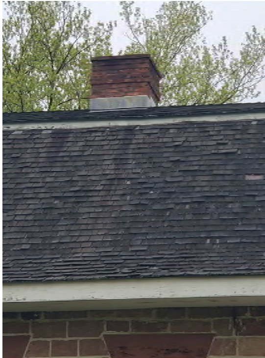
DETERIORATED CEDAR ROOFING
