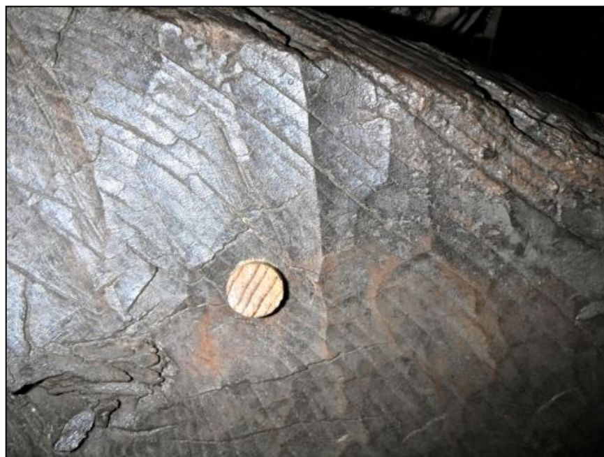
Figure 5: Detail of Core Sample Location and Plug
