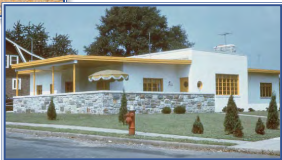
HACKENSACK HOUSE/STUDIO CA 1958. UNFORTUNATELY, THIS BUILDING IS NO LONGER EXTANT; IT WAS DEMOLISHED SHORTLY AFTER ITS SALE IN 1987. A DOCTOR'S OFFICE NOW STANDS ON THIS SITE AT THE CORNER OF PROSPECT AND THOMPSON STREETS. -VAN GELDER PHOTO ARCHIVE
