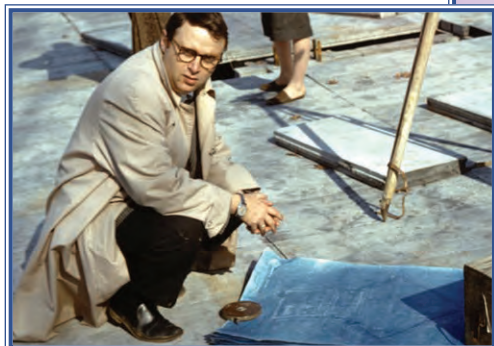
RUDY VAN GELDER PORING OVER THE BLUEPRINTS AT THE ENGLEWOOD CLIFFS CONSTRUCTION SITE. -VAN GELDER PHOTO ARCHIVES
