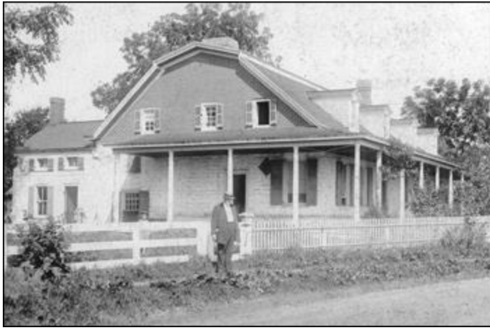
D. Anderson Zabriskie, last private owner of the Steuben House
